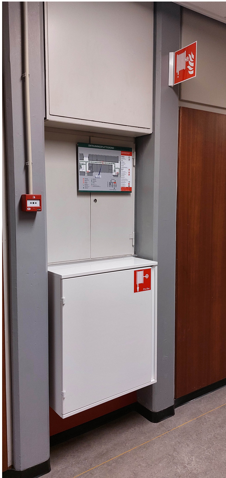
Figure 9: * At several places one clearly indicated signs of fire extinguishers, and alarms.
